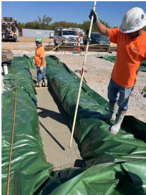
Vapor barrier and mud sill install beneath the trench drains at the App Bay
